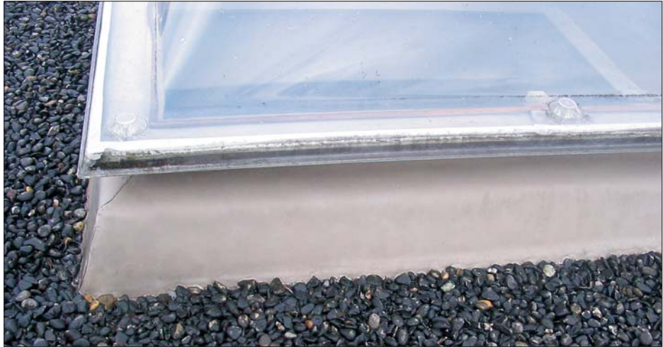
Fig. 4: Flashing at skylight, roof of Brunner building in Flawil (Switzerland)
