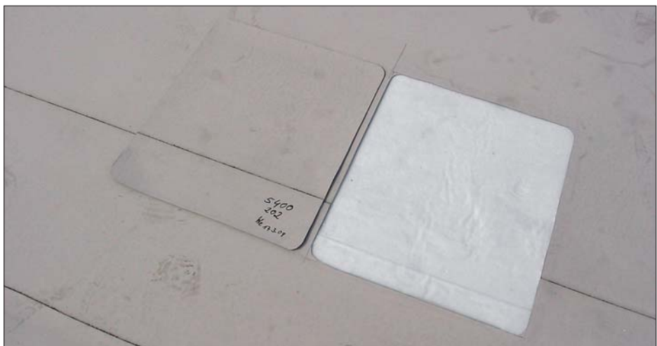
Fig. 6: Sampling on the roof, Tries building in Ehingen (Germany)
