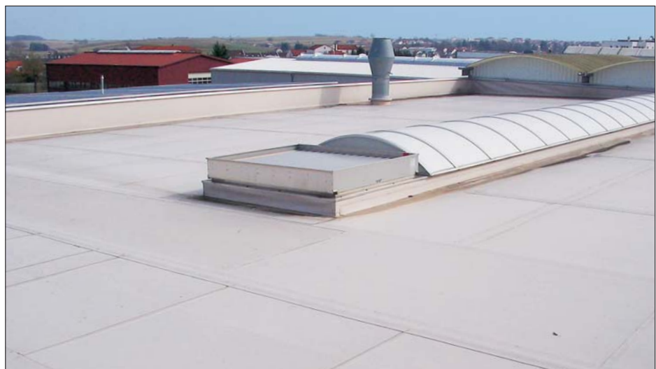
Fig. 3: Overall view of roof, project Tries in Ehingen (Germany)
