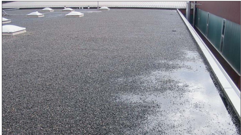
Fig. 2: Overall view of roof, project Brunner in Flawil (Switzerland)
